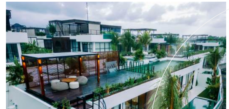
● GARDEN VILLA II 4 units Project area 1.607 sq.m. Construction area 455 sq.m.
